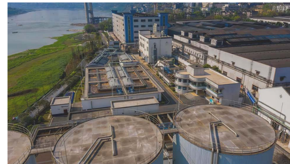
Panorama of Luohan Brewing Ecological Park Wastewater Treatment Station
