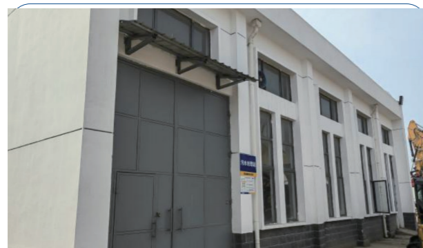
Waste water treatment station
