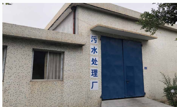
Shihushan Terminal No. 1 Sewage Treatment Plant
